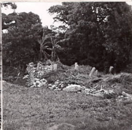
Bomb damaged Ruins
