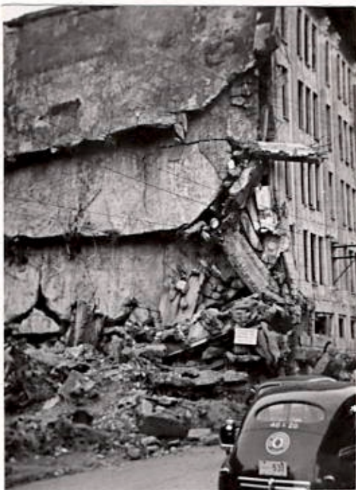
Damaged Building in Manila
