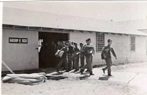
Issuance of supplies
